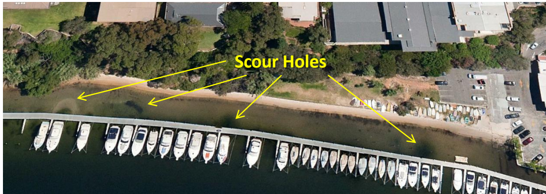
Figure 34: Scour holes caused by vessels in yacht club pens
