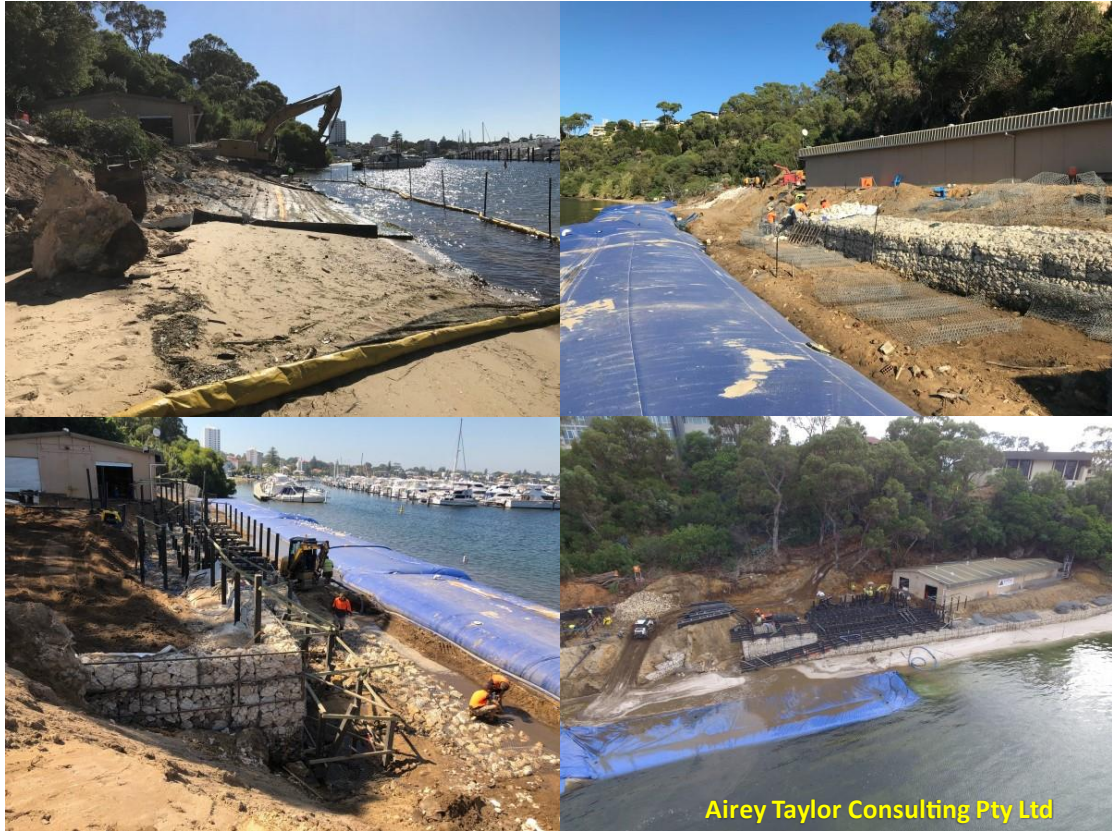
Figure 36: Reconstruction Works at Christchurch Rowing Shed
