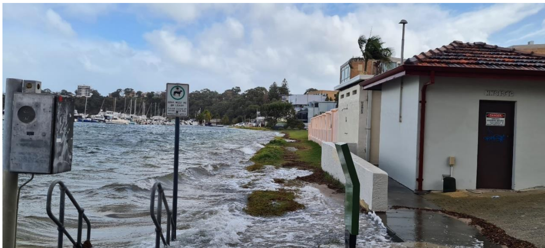
Figure 45: High water levels on 25 May 2020 - looking west from Claremont Jetty
