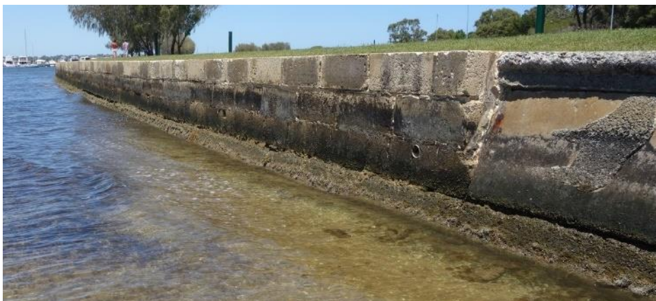
Figure 7-12: Section of new vertical limestone block walling constructed on existing footings
