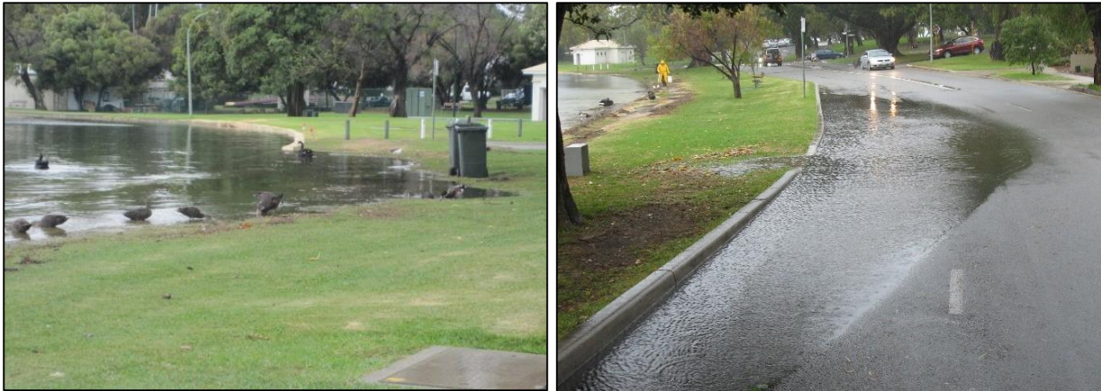
Figure 9-18: Inundation and Surface Runoff Ponding during 20 May 2011 Storm (Source: SoPG)
