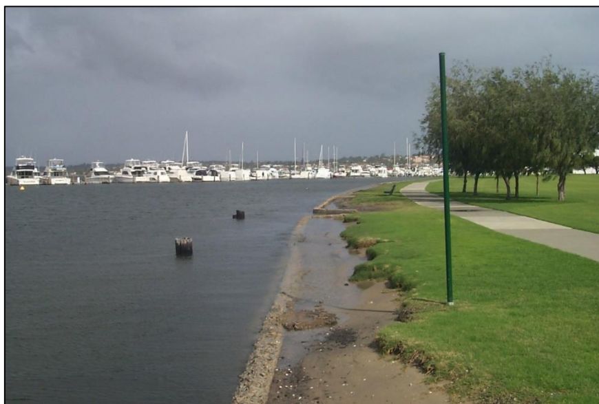
Figure 12-7: Inundation at Charles Court Reserve 16 May 2003
