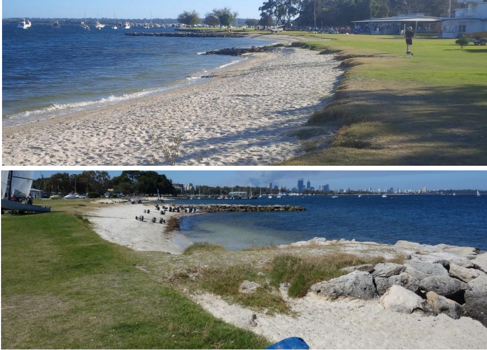
Figure 7-10: NYC with groynes and beaches riverward of old walling
