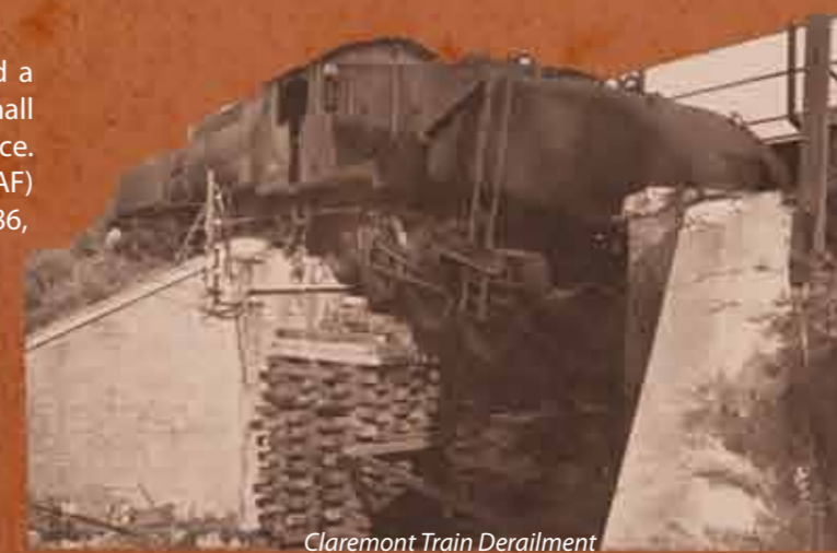
Claremont Train Derailed
